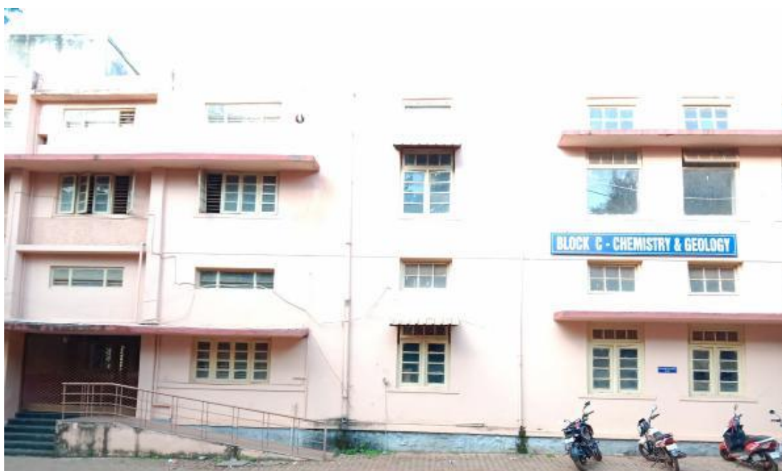
Picture of the building of Karnatak Science College, Dharwad, which houses the Principal's Chamber, Office, UG & PG Department of Chemistry, the Statistics Lecture Hall and the Department of Geology KSCD
